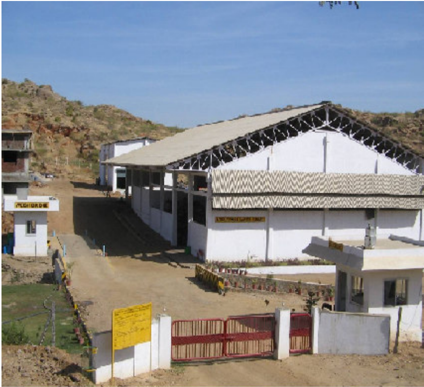
HAZARDOUS WASTE TREATMENT PLANT
